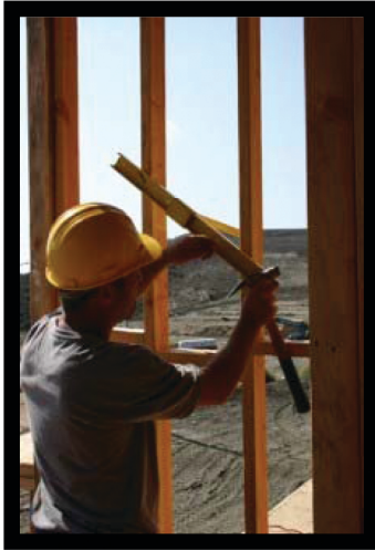
1. Attach Spanner Bracket to framing members using two 16 duplex nails.
